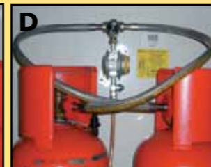
Picture shows a Truma regulator upgraded to a manual changeover with a 01-1630 and using two propane 0.75 meter Stainless hoses. Note how the hoses cross preventing unnecessary kinking and twisting.
